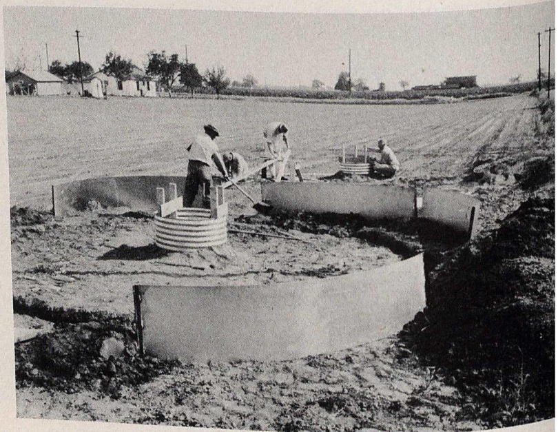
FIGURE 13. Digging trench for dike
