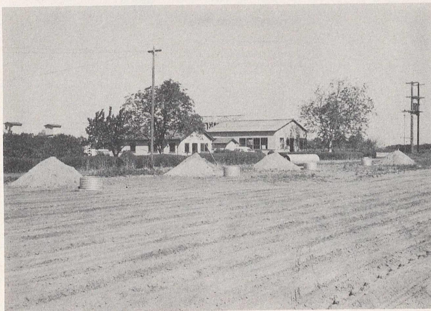
FIGURE 4. Sampling wells in place
