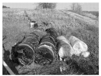
Picture 24: Woodbury Site – Close up of Asbestos Bags & ACP Pipe Staged for Loading (11/18/2009 Photo by William Westley Approved by Mark Hostrawser).
