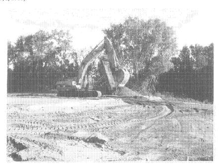
Photograph 24: D9 Staging Area – Bolander Generates Stockpiles on the EW-1 Stockpile Staging Area from the Excavated D9 1-9 Soil Block (7/2/2010).
