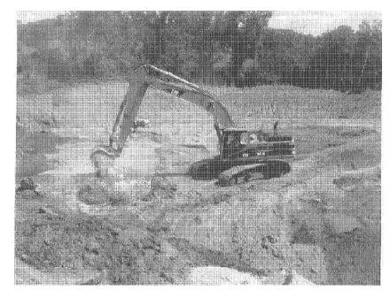
Photograph 9: D9 Area – Bolander Mixes 10 Bags of LKD Into Soil Block D9 2-7 to Stabilize Soils and Support Heavy Equipment (7/26/2010).
