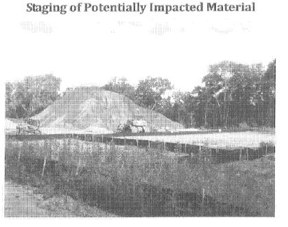
Photograph 20: D9 Staging Area – Potentially Impacted Material Staged on PIM-1 maintained with Dedicated Dozer (6/22/2010).
