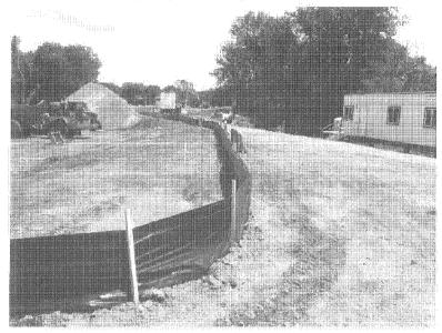
Photograph 19: D9 Area – Installed Silt Fence along South Side of D9 with Top-of-Slope Staking on Interior (6/3/2010).
