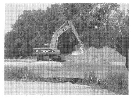
Photograph 8: D9 Staging Area - Bolander Mixing LKD into the D9 1-9 Stockpiles for Onsite Conditioning (7/20/2010).
