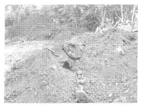
Photograph 32: D9 Staging Area – Encountered Empty Crushed Drum Fragments from Potentially Impacted Material (6/10/2010).
