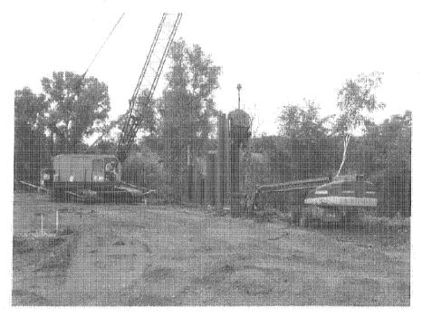
Photograph 4: D9 Area – Sheet Piling Early Refusal along East End of Wall Due to C&D Waste along Slope (6/2/2010).
