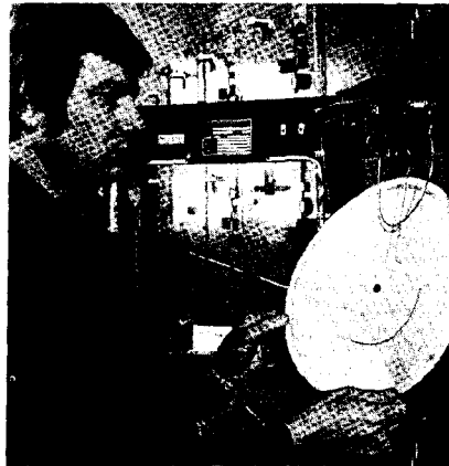
Jeff Duviea checks a recorder which monitors the Company's wastewater treatment plant at Chemolite. The plant treats about 5 million gallons of water a day and removes more than 95 percent of the wastes from the water.
