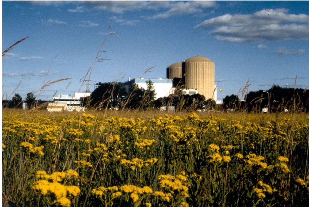
Prairie Island Nuclear Generating Plant, Units 1 and 2
