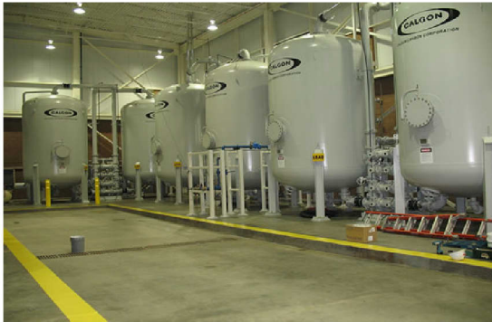
Image: City of Oakdale water treatment plant
