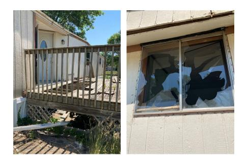
As the photos of this property show, one entire side of the home has no siding and there is a hole in the upper right corner of the home. The home is missing much of its skirting, leaving the area underneath—which contains debris and electrical cords—exposed. The porch is missing boards, creating a large gap in its floor. Many of the home's windows are broken with jagged shards of glass remaining.
