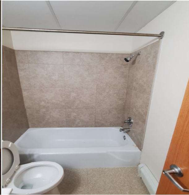
Clean move out condition of Bathroom
